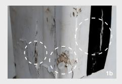
(1b) Indicates visual signs of impact damage on the corner of the column, note the patch of vinyl missing in the impact area, and the splitting in the vinyl where the column has delaminated. Any stand displaying this type of damage SHALL NOT be used.
